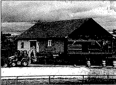
Canal freight house moves to its new location.
