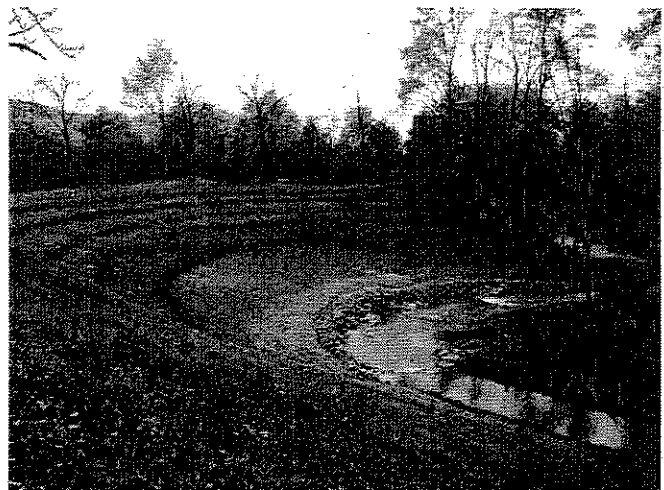
After Construction - In-stream Structures and Soil Bioengineering.
