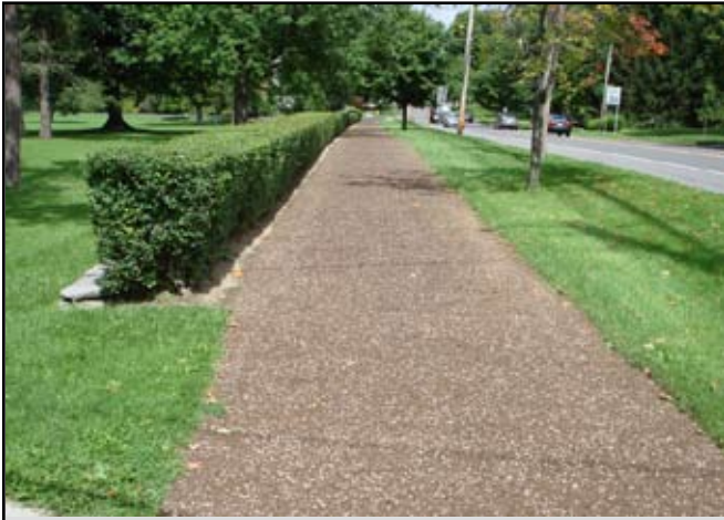
Figure 3-4. Green infrastructure: An example of porous pavement. (Source: Central New York Regional Planning & Development Board)
