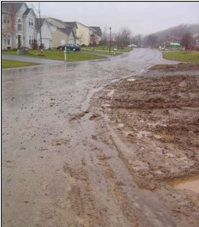
Figure 3-19. Runoff from construction sites with poor erosion control carries sediment and nutrients into municipal drainage systems and to Onondaga Lake. This is a major cause of non-point source pollution. Efforts to educate the construction industry about these impacts continue. (Source: Central New York Regional Planning & Development Board)
