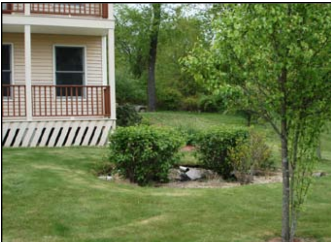
Figure 3-3. Example of a rain garden, a form of green infrastructure. The white pipe observed between the two shrubs is a downspout from the roof of the adjacent building. (Source: Central New York Regional Planning & Development Board)
