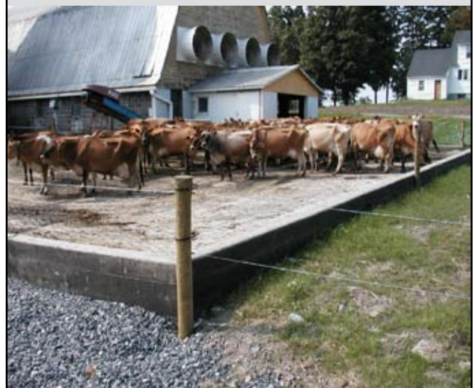
Figure 3-17. Post-BMP barnyard with concrete pad to reduce erosion and enhance animal waste management. (Source: OCSWCD)
