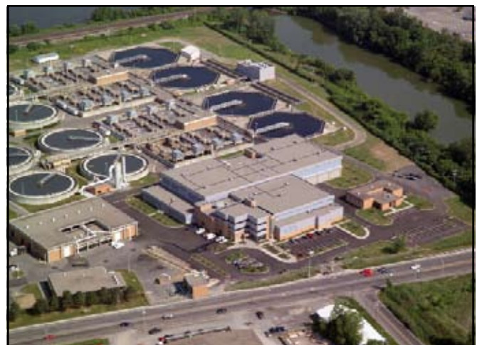
Figure 2-2. Aerial view of new facility at METRO. (Source: OCDWEP)
