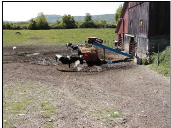
Figure 2-20. Pre-BMP barnyard at a farm in Onondaga County. Soil erosion and surface runoff of nutrients from barnyard can pollute streams. (Source: OCSWCD)
