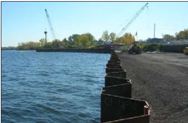
Figure 2-7. Barrier wall installation. (Source: NYSDEC)
