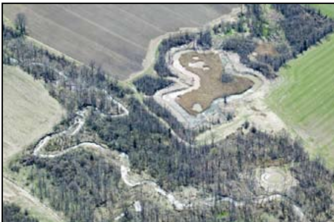
Figure 2-12. Aerial photo of mudboils and impoundment dam alongside Onondaga Creek. (Source: USGS)
