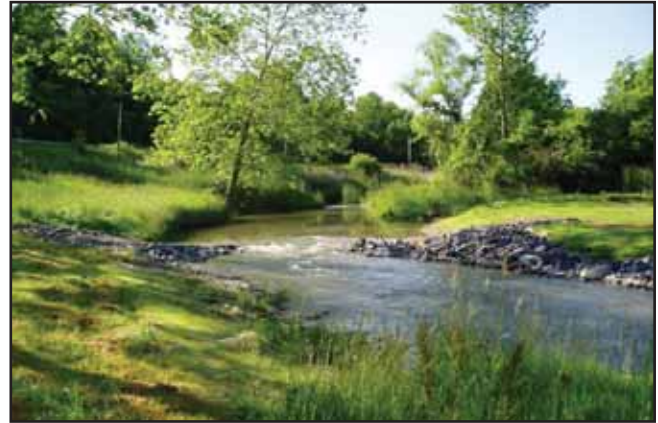
After: Creek erosion prevention project using crossvane weir technique in center.
