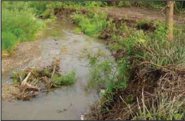
Before: Onondaga Creek right bank erosion prior to restoration.
