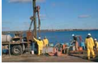
Installation of wells to intercept contaminated groundwater along lake shore
