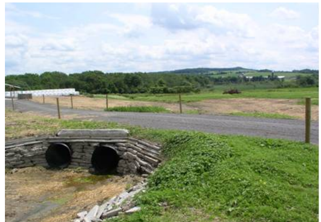
After – Stream crossing installed with livestock laneway for pasture access.
