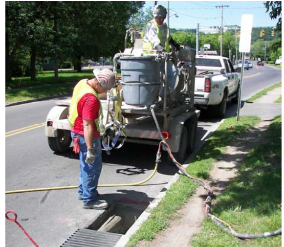
Catch Basin Rehabilitation Equipment
