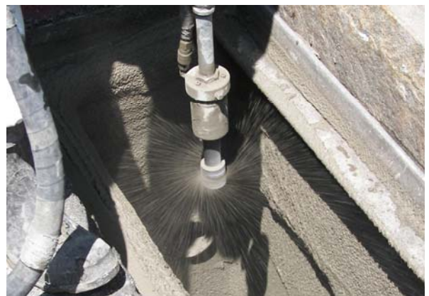
Cementitious Lining Being Applied to Catch Basin
