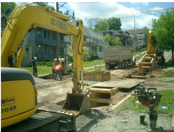
Sewer Separation Construction
