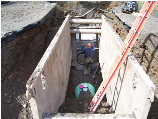
Manhole and Pipe Installation
