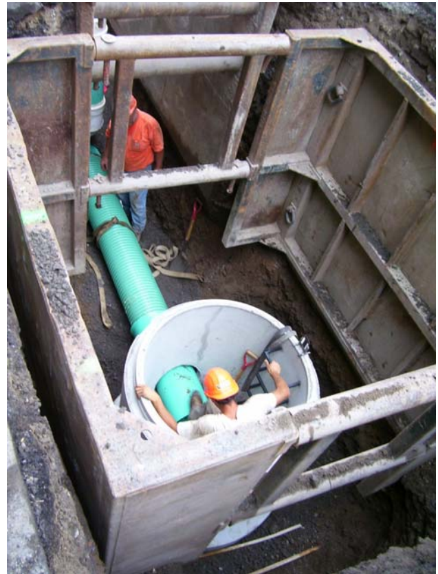
Manhole Installation
