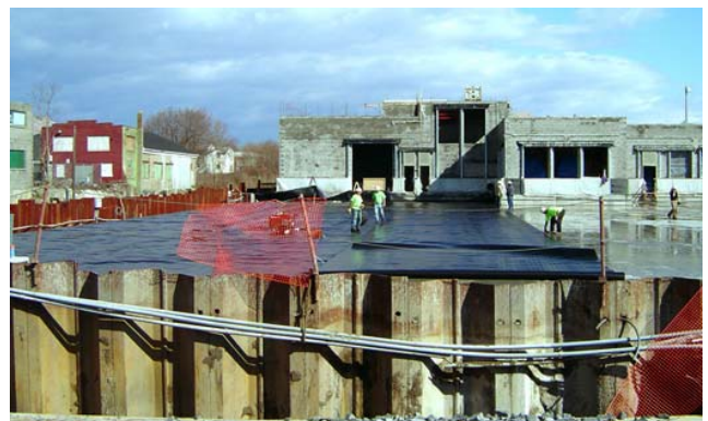
Roof Liner on Underground Storage Tank
